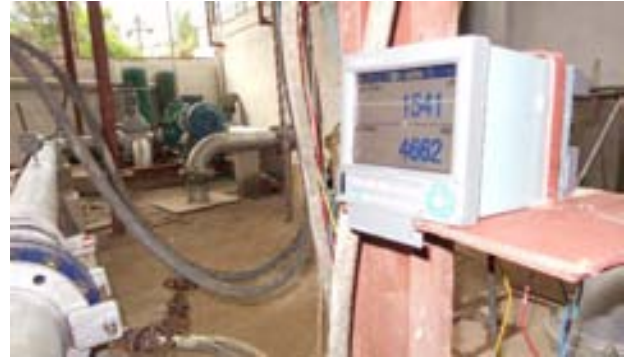
Online chartless recorder for HMI system converting analog reading results for online pressure and flow changing results
